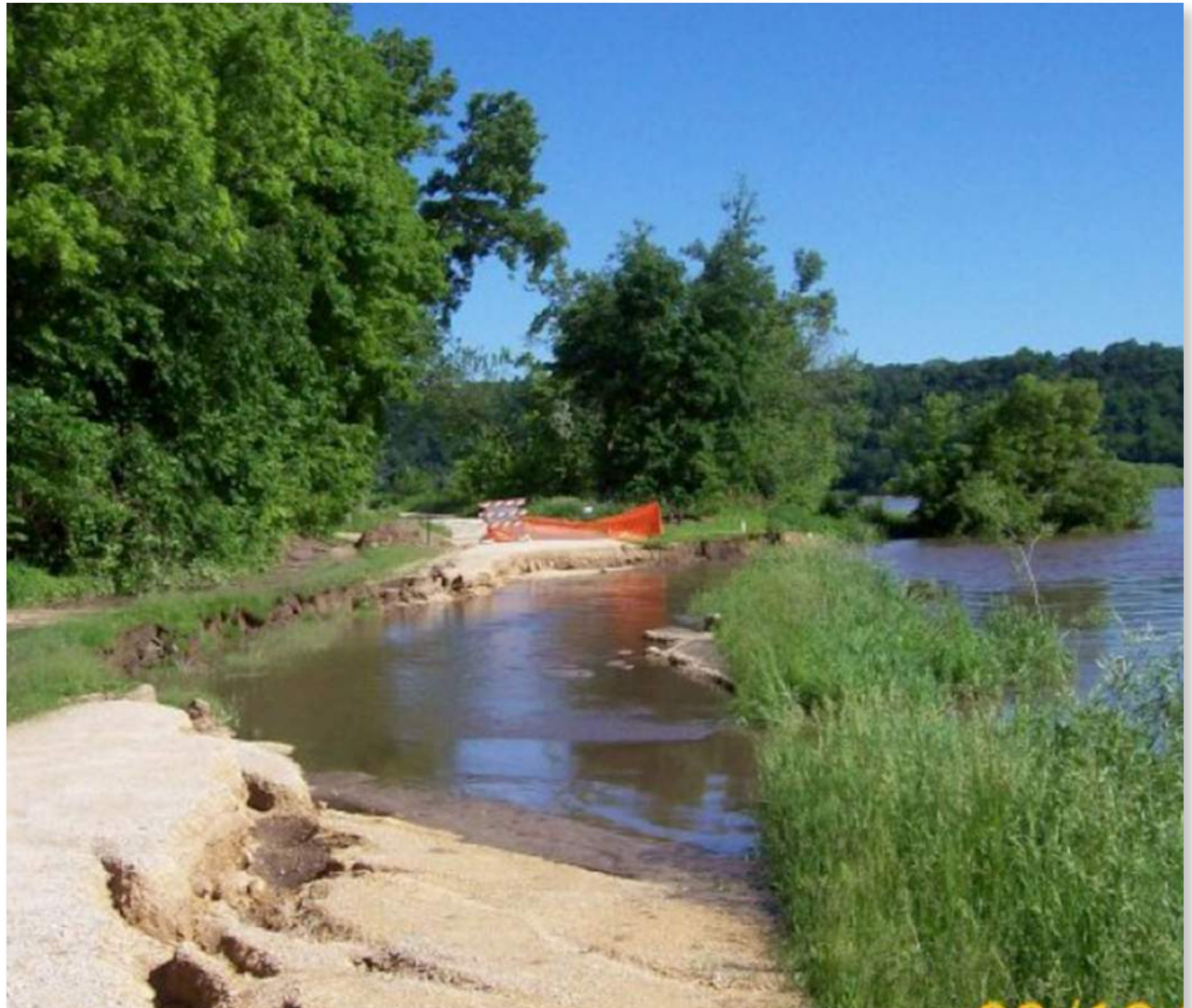
Infrastructure Damage in the TRW
