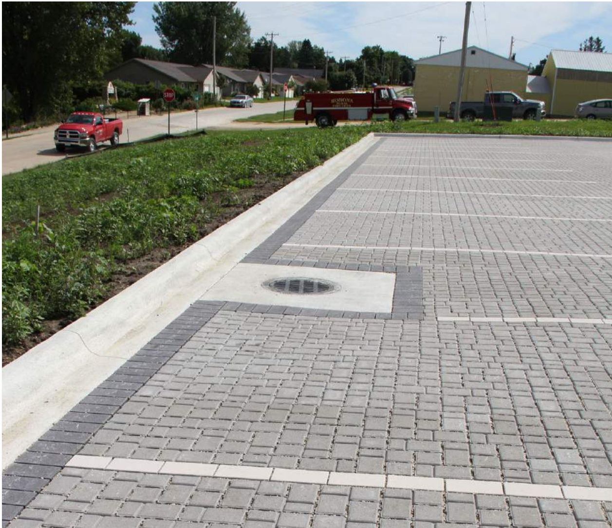
Several TRW Communities are Planning to Install Permeable Pavers
