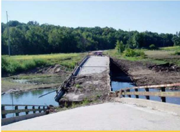
Fayette County Bridge Destroyed in Flood Event
