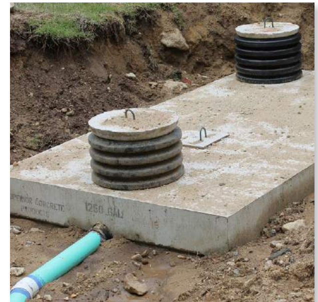
Septic System Replacement
