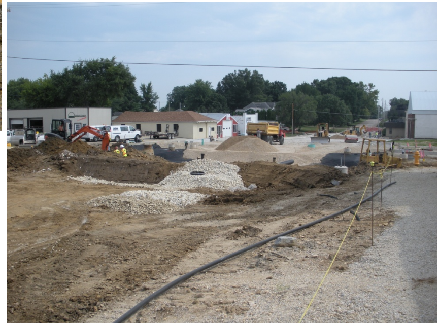
Sediment Berm With Inlet & Crushed Stone Filter
